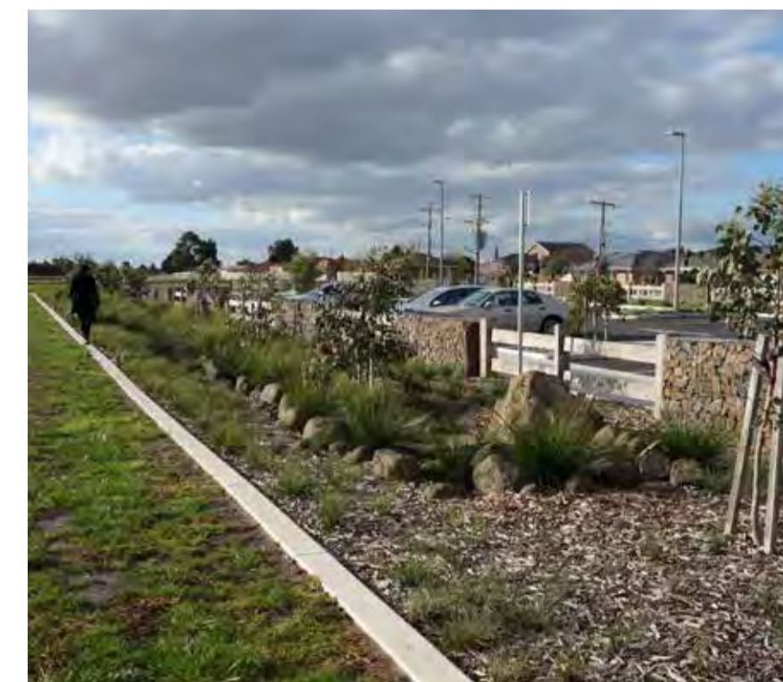
New consolidated car park with associated planting and water sensitive urban design treatment systems
