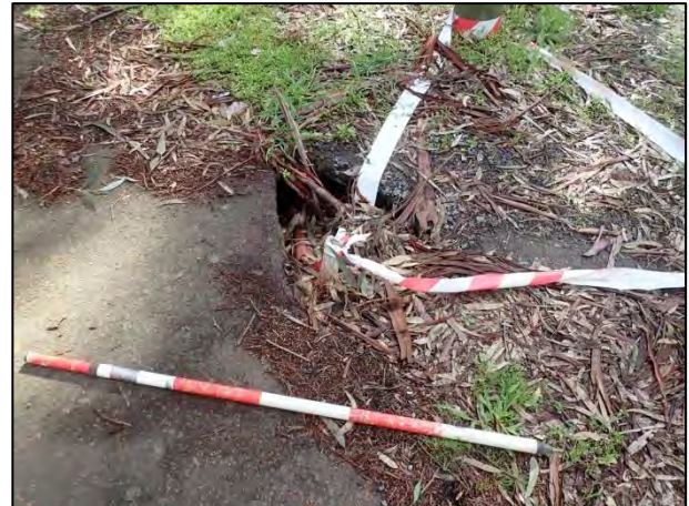
Plate 4: View of sinkhole along northern edge of Yarra Flats Entry Road (photo by S. Anderson 03/09/2018)
