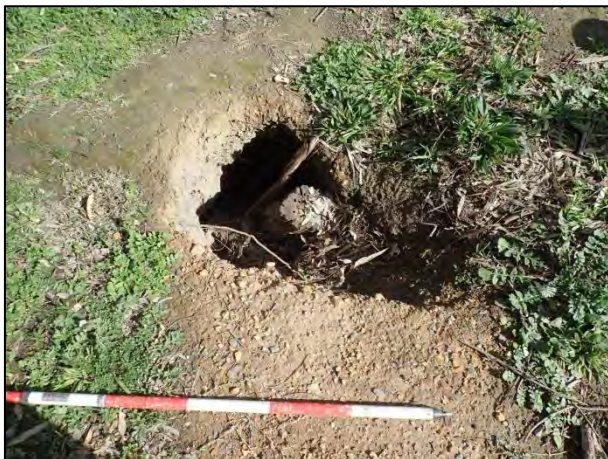
Plate 5: View of sinkhole along northern edge of Yarra Flats Entry Road (photo by S. Anderson 03/09/2018)
