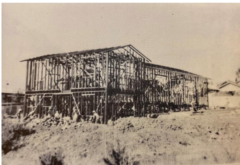
Timber frame, awaiting cladding, 1939 (Source: Brooks, 2 nd Ivanhoe , p35)
