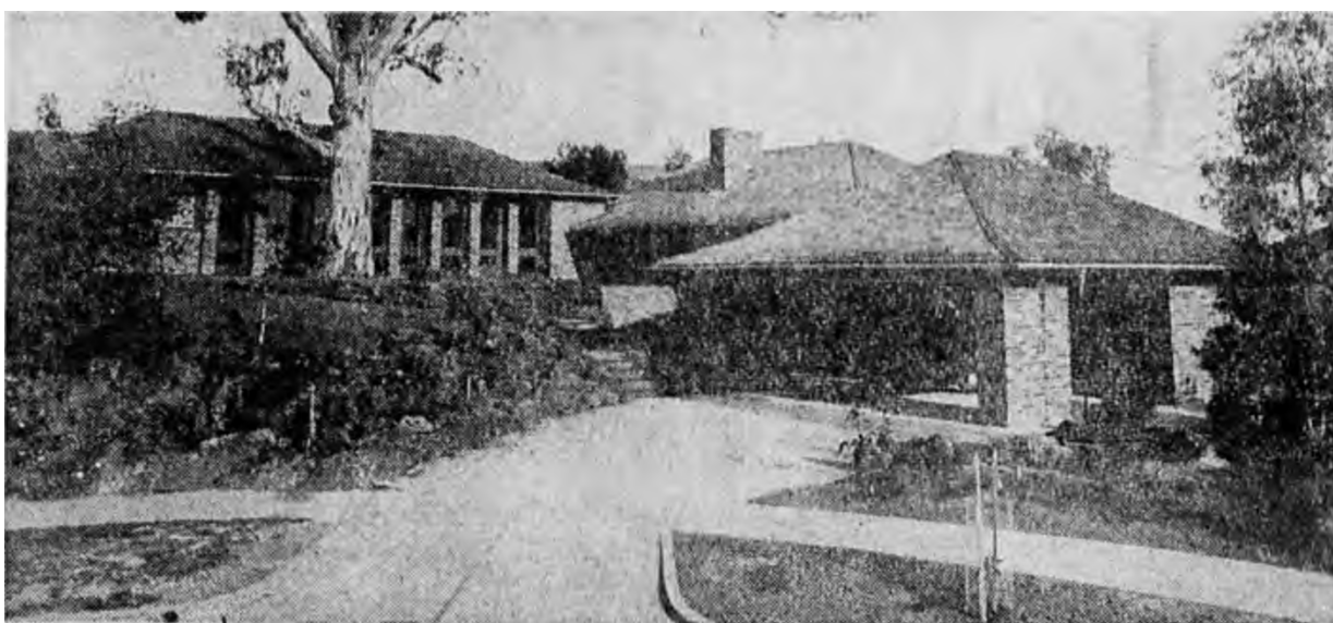
'Three different floor levels with separate roofs allow a logical group of sleeping, living and car accommodation of this impressive Heidelberg home.' (Source: Baker, Barker, Age , 11 December 1972, p14)
