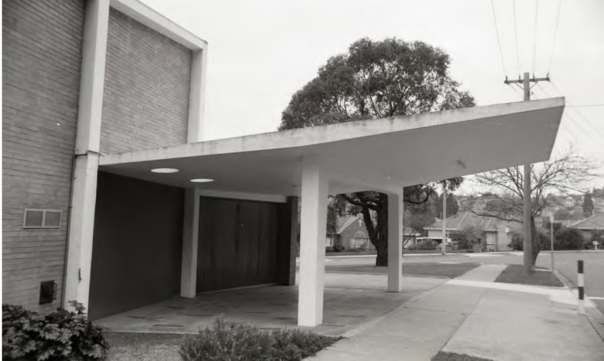
Close-up of cantilevered porch, mid-1980s – soon after partly enclosed with glazing, mid-1980s Note original floor of white Carborundum (silicon carbide stone) panels and 'English' grey-blue quarry tiles The mature tree central to the triangular front garden (background) has since been replaced (Source: courtesy of Graeme Butler)
