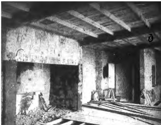
'Roof and floor construction shows in this progress shot.' (Source: Johnston, 'Built from the good earth', AHB June 1948, p29)
