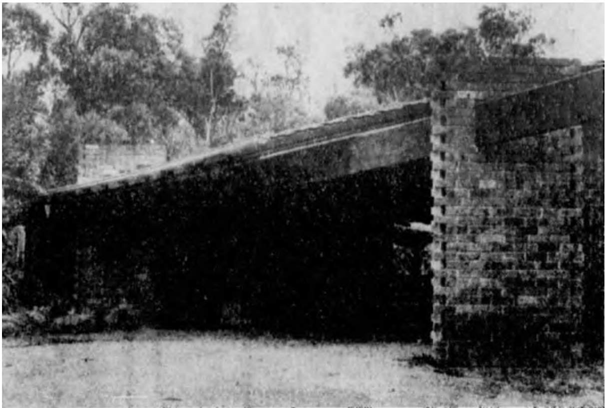
'Heavy laminated beams supported on brick piers enclose the carport of Charles Duncan's design at Lower Eltham' (Source: Barker, "The Age" — RAlA Citation Award No. 34', Age , 15 May 1972, p11)
