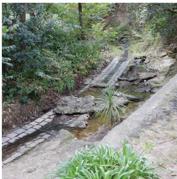
Figure 33 - Damaged bluestone lining to Salt Creek
