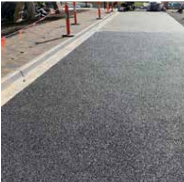
Porous Lane Permeable pavement system at tree base - tree pit
