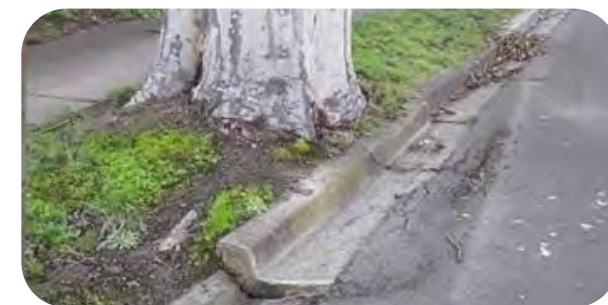
Figure 11. Poor soil depth, small planting footprint and compacted soils cause damage to footpaths. Source: Banyule City Council
