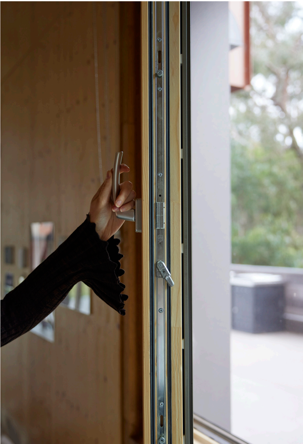
High-performance double-glazed, thermally broken windows. Photography by Kim Landy.
