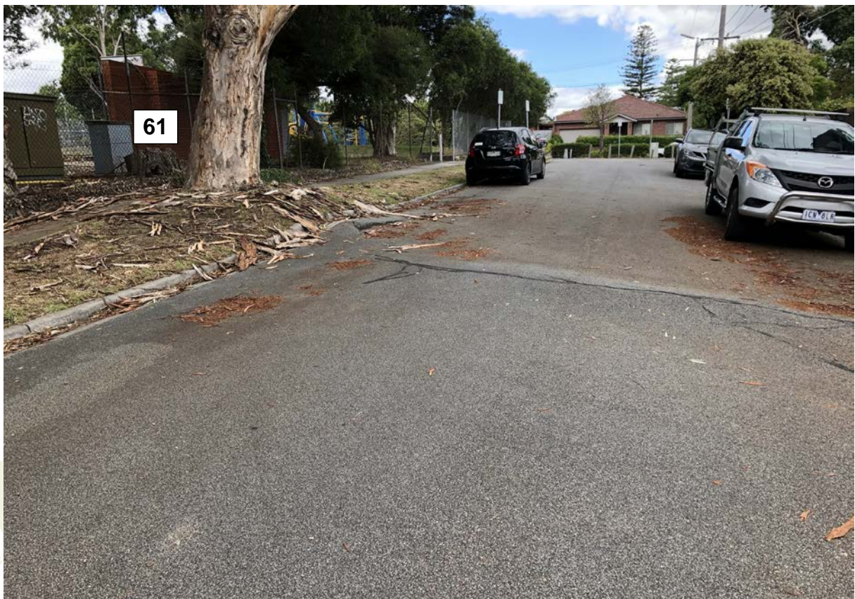
Image 19: Base of Tree 61 facing east, showing longitudinal damage to road surface and repairs. Appropriate TPZ fencing must be established and maintained for the duration of site works. Any alteration to the existing site conditions must be based on arboricultural advice and subject to arborist supervision to ensure no damage occurs to roots, buttress, trunk and limbs.
