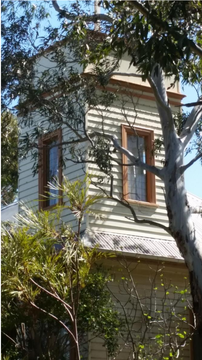
Figure 16. Detail of the prominent and unusual tower, showing solid balustrade, notched weatherboards to the topmost panels, the projecting hip roof at the base of the first floor, and timber-framed louvre windows with moulded architraves and sills. (Source: Context, September 2018)
