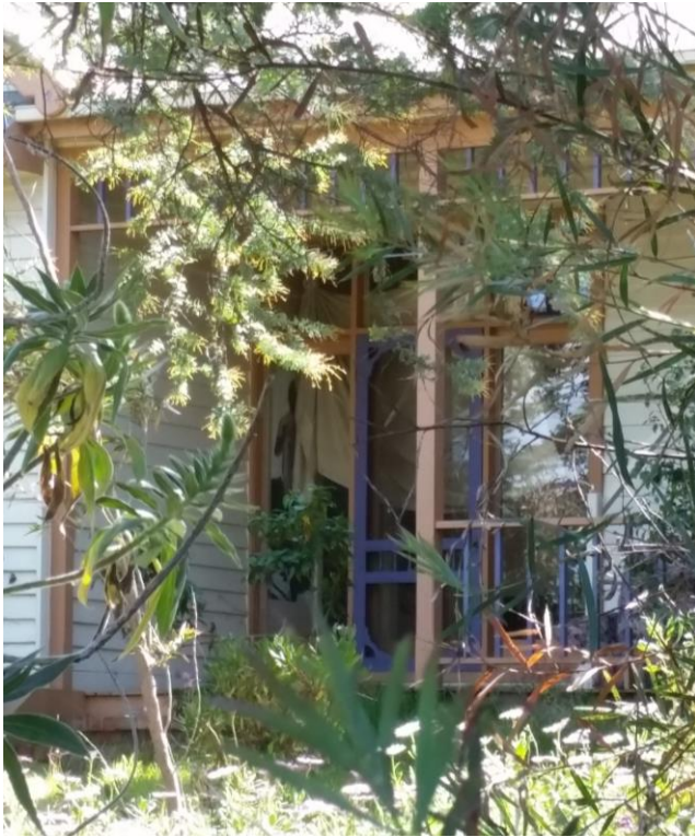
Figure 17. Detail of entry porch at the south elevation showing simple timber fretwork and balustrade, early timber door frame enclosed by later side and highlights. (Source: Context, September 2018)
