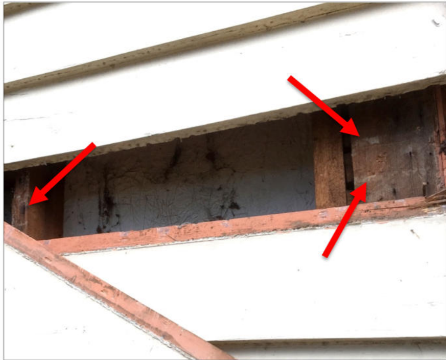
Figure 18 Detail of the front elevation with a weatherboard removed. The exposed studs have markings consistent with horizontal laths, over which roughcast render would have been applied.
