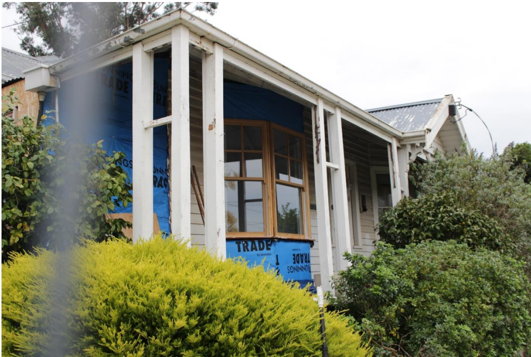
North-west corner, showing where window has been removed and (blue sheeting) and replaced multi-paned upper sashes to northern bay of façade. Not the frieze and other decorative elements between the posts to the verandah have been removed.
