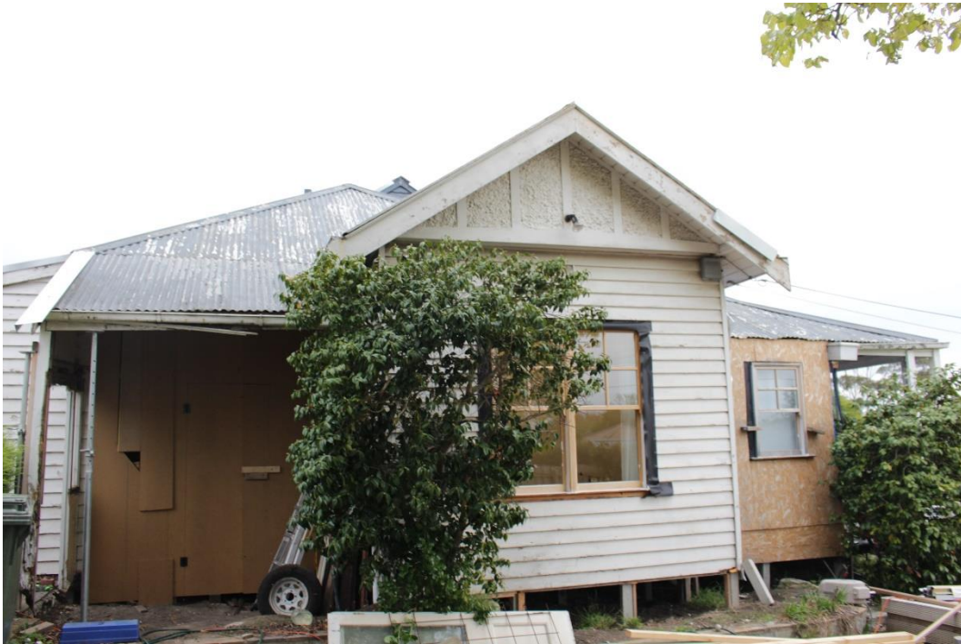
North elevation – altered window at west end and new multi-paned upper sashes below gable end
