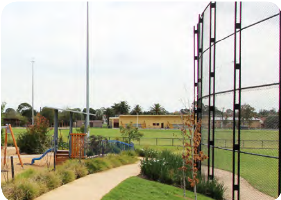
Example of chain wire ball catch fence
