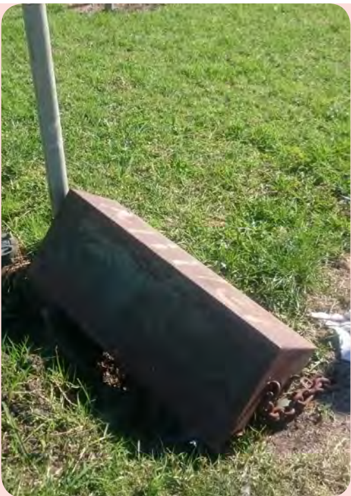
Park water meter enclosures damaged
