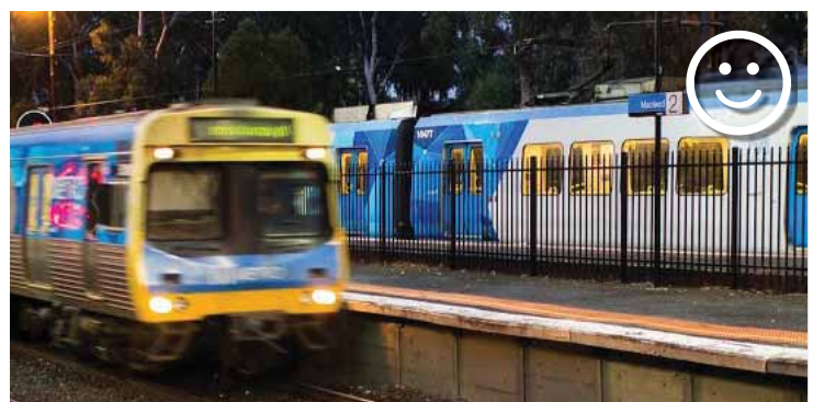
good example of recessive fencing to station
