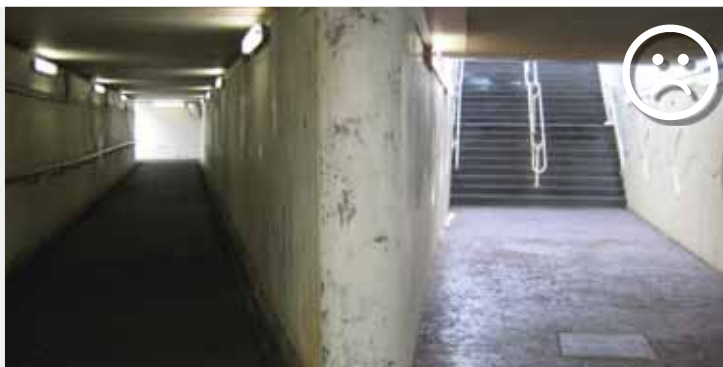
poor example of visual connectivity throughout station
