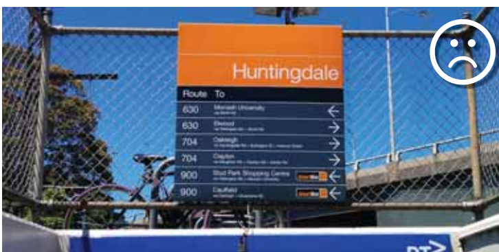
poor example of fencing to station platform
