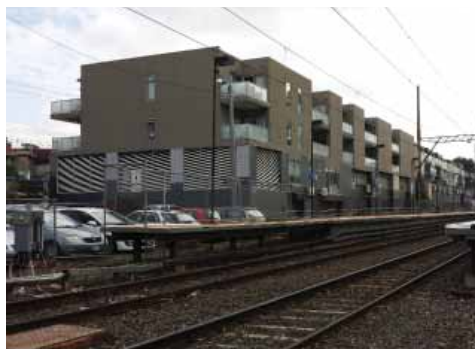
existing commuter car parking at station
