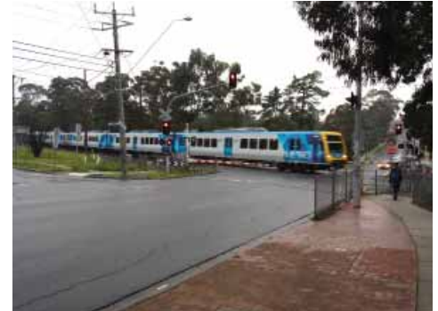
existing condition of level crossing at station
