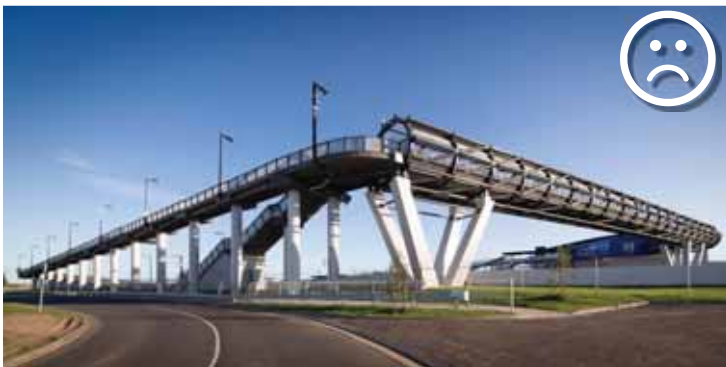
poor example of efficient station entry
