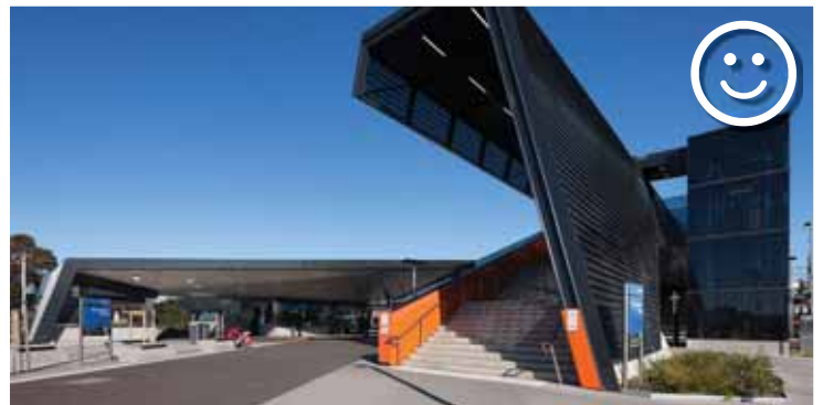
good example of multiple access points to station entry
