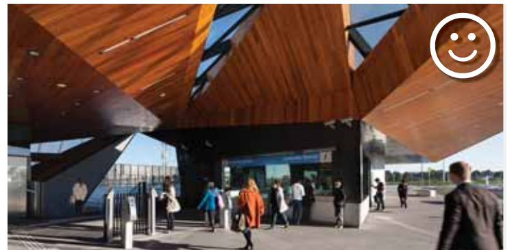
good example of a resilient station building allowing for future technology adaption
