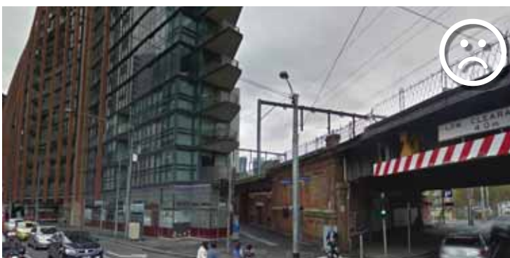
poor example of apartment interface to elevated rail corridor
