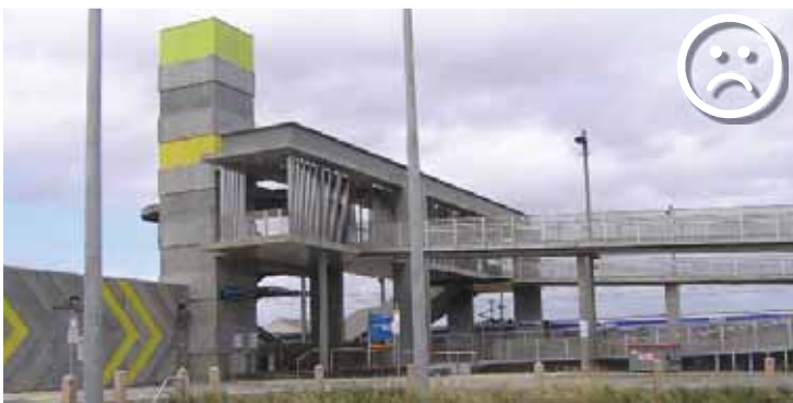
poor example of station building entry to the public realm
