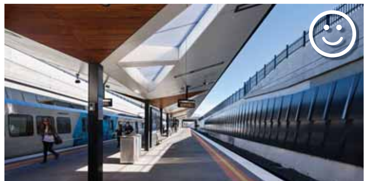
good example of daylight access and shelter to station platform
