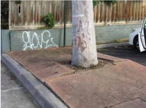
existing conditions of pavement in Rosanna Village
