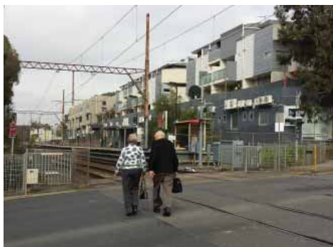
existing level crossing conditions north of station
