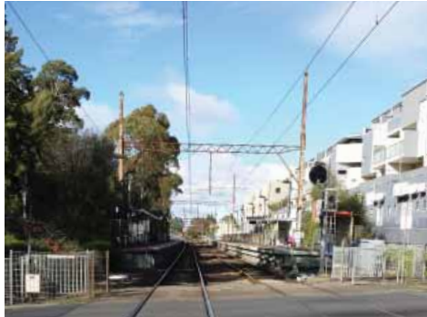
view of station platforms from level crossing
