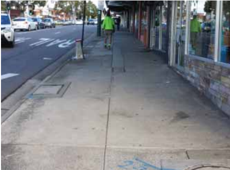
existing conditions of footpath within village
