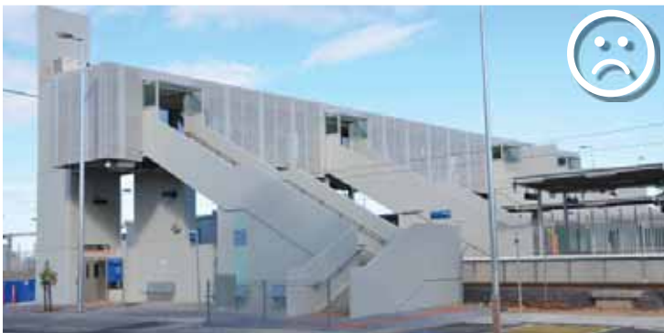
poor example of a train station interface to the public realm
