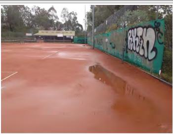
There is a grated pit in the north eastern corner of the enclosure. This court surface would be expected to drain through the surface, although it appears to be compacted in places, causing water to pool along the surface. This is particularly the case at the northern end of the enclosure, where extensive
